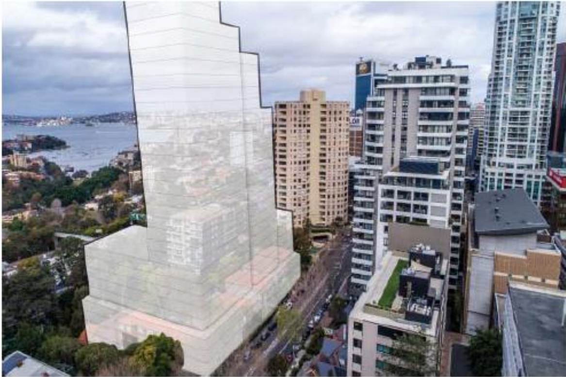
Figure 19 - View from the north east at 168 McLaren St (Source: VIA)
