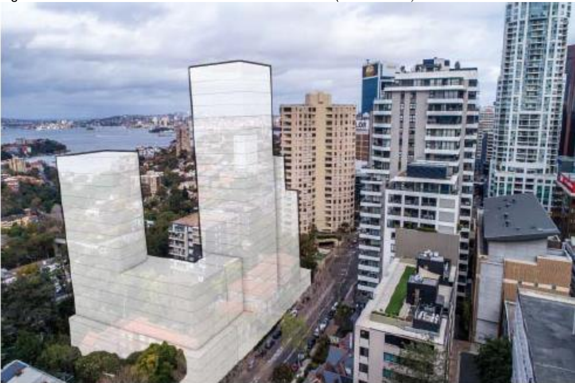
Figure 20 - View from the north east at 168 McLaren St (Source: VIA)
